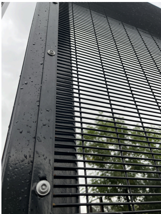
Clamp bar and security fixing detail
