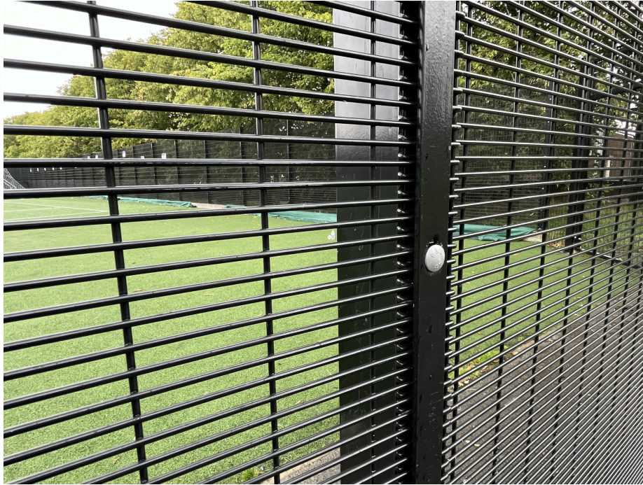
Continuous clamp bar and mesh connection
