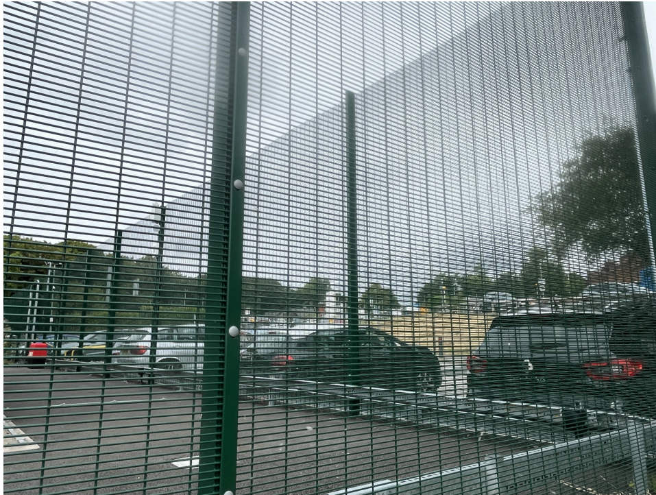
358 mesh and post installation
