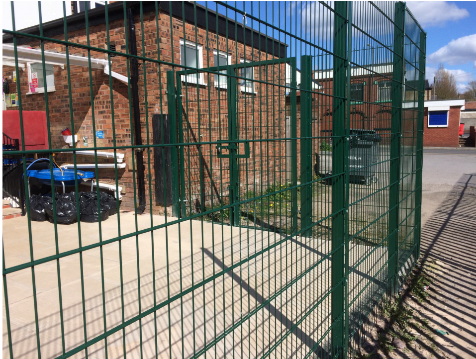
868 twin wire mesh installation
